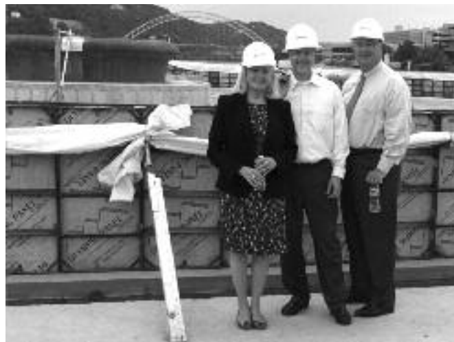
Above: Visiting the fountain's construction site: Lisa Schroeder, President and CEO of Riverlife; Grant Oliphant, President and CEO of The Pittsburgh Foundation and chair of Riverlife's Board; and Jim Rohr, Chairman and CEO of PNC, a partner on the Three Rivers Park development project.
